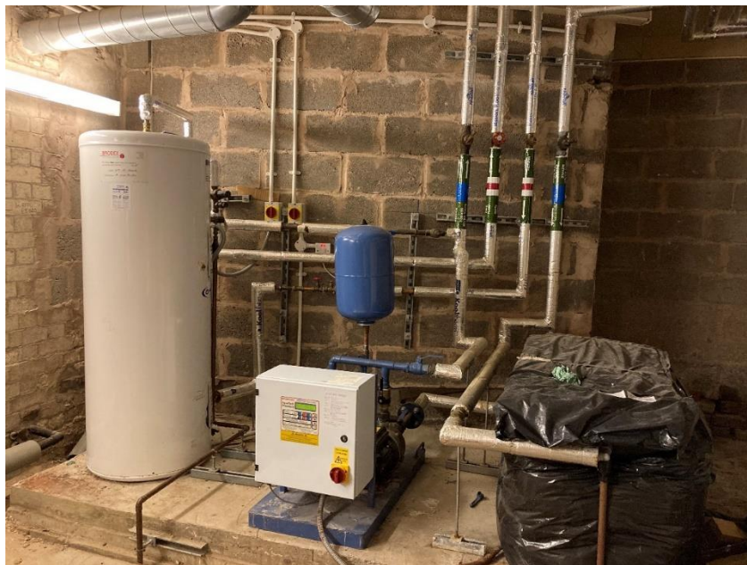
Figure 6 – Domestic Hot Water (DHW) system.
