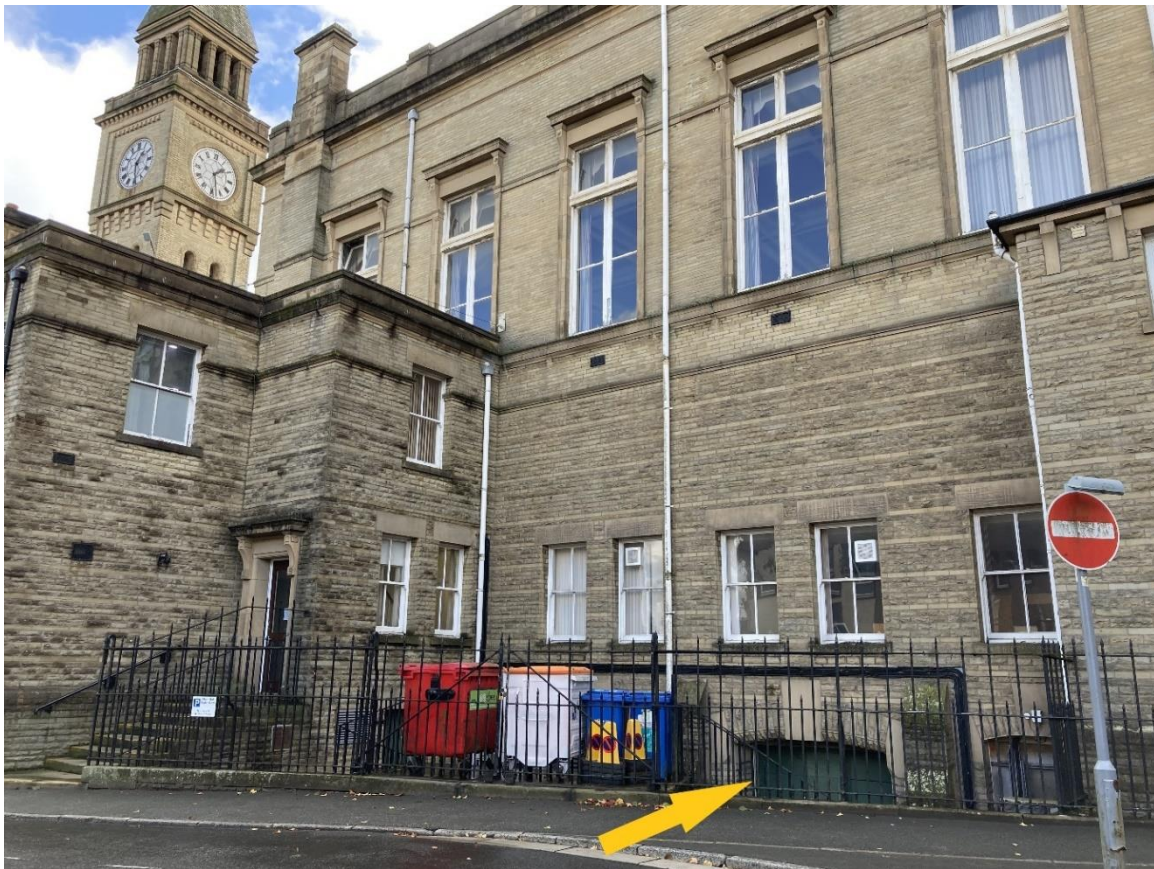
Figure 3 – Town Hall entrance to basement from Mealhouse Ln.
